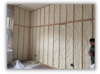
Once the foam was up, the wallboard went in and the walls were painted. Mini-split heat pumps were installed in these rooms for AC and heat. This will allow the temperature to be independently controlled in each room to accommodate the needs of different activities and the demographics of the participants. The old radiators are still in place but will hopefully go on infrequently.
